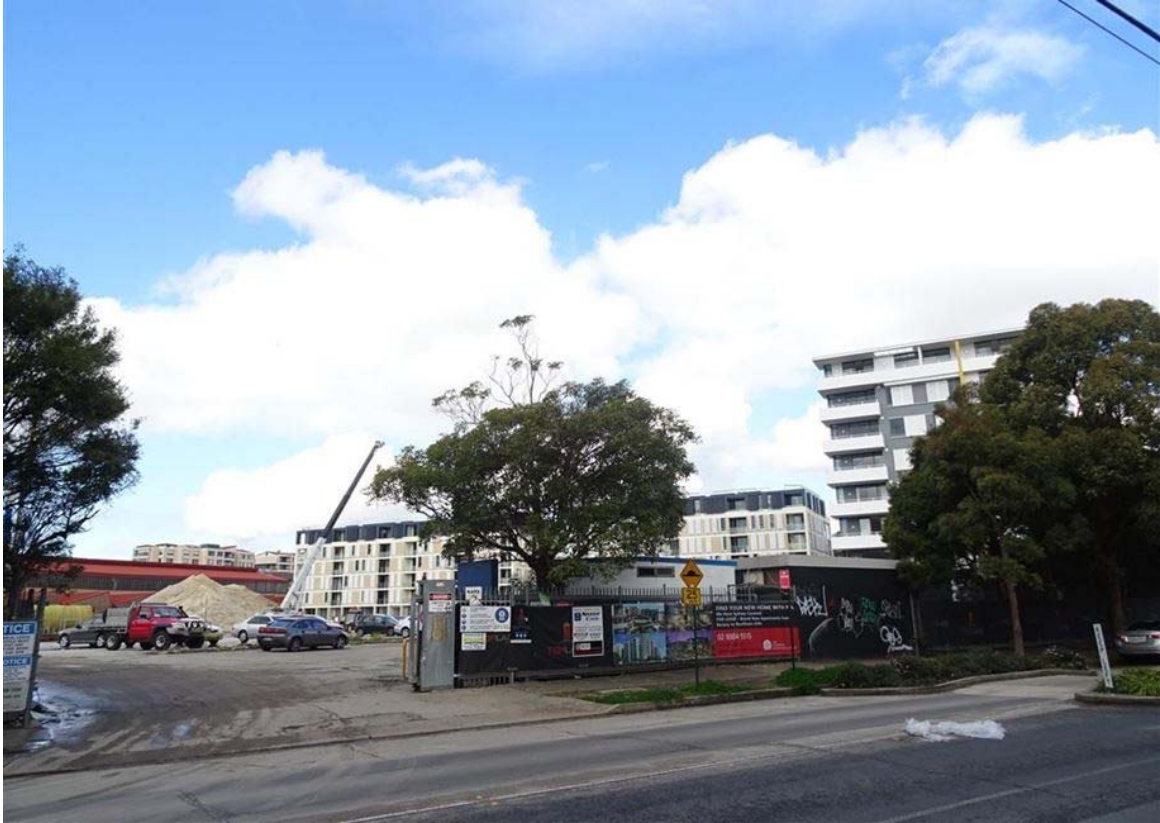
Figure 4: The site viewed from Dalmeny Avenue.
