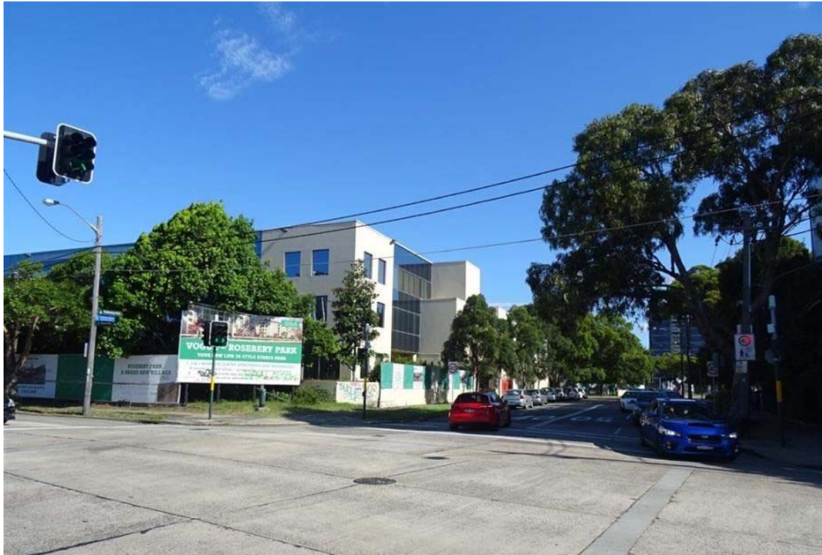
Figure 3: The northern end of the site viewed from the corner of Epsom Road and Dalmeny Avenue.
