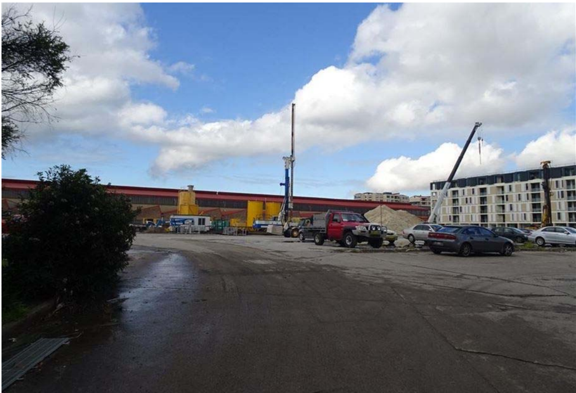
Figure 5: Looking east across the site.
